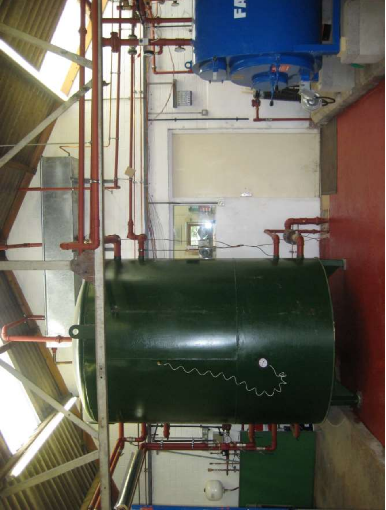
Boiler and 2000 gallon (9000 litre) accumulator installation, prior to insulation at FARM2000, Bradley Green, Redditch
